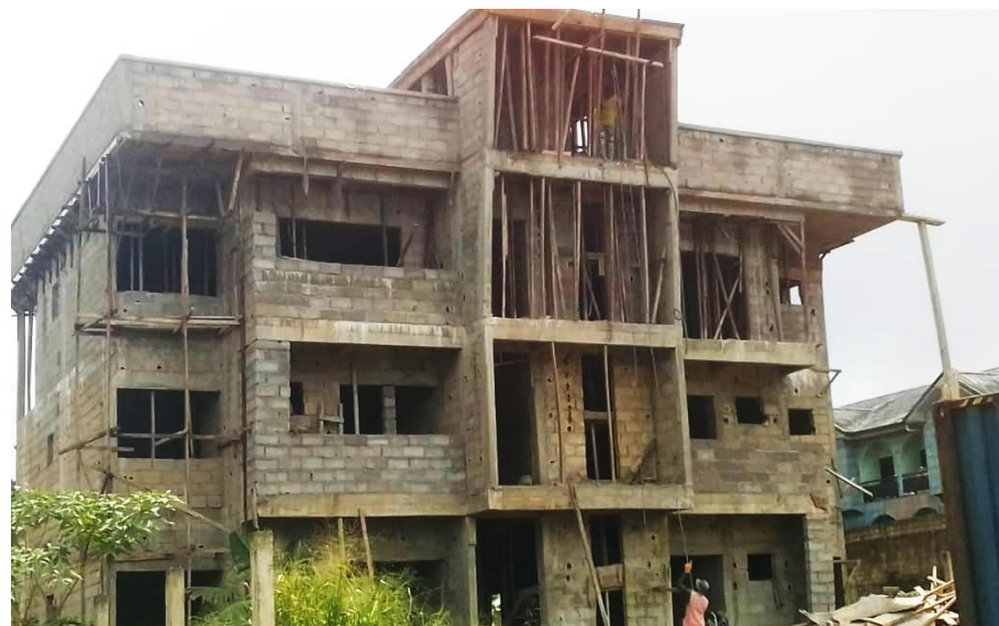
Chantier - BLAISE T. BUILDING
